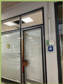
Janitors' room: on the right side of the entrance. lost items are kept there to be picked up
